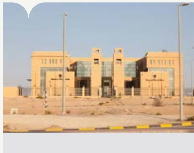
Al Muzeerea Police Station in Liwa Client: OTIS Brand: OTIS | Quantity: 08
