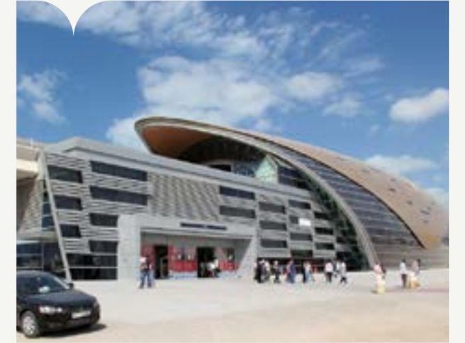
Metro R13 T1T2 Client: Al Yousuf Electronics LLC Brand: Fujitec | Quantity: 02
