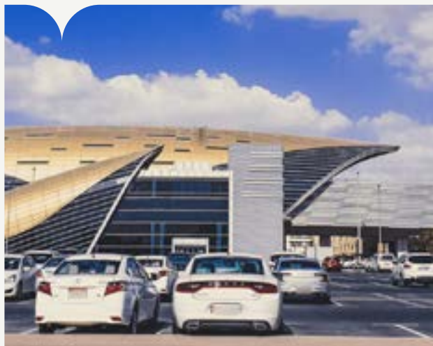
Metro Green Line Client: Al Yousuf Electronics LLC Brand: Fujitec | Quantity: 08
