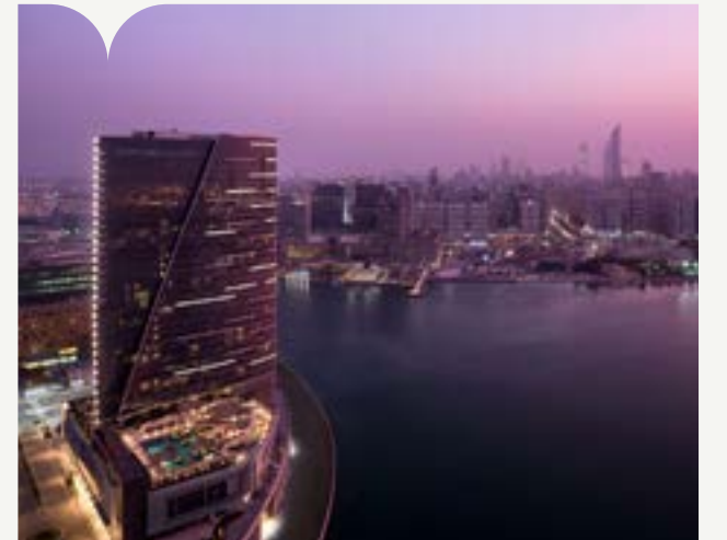
Rose Wood Hotel - B Client: ThyssenKrupp Brand: ThyssenKrupp | Quantity: 04
