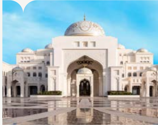
Presidential Palace Abu Dhabi Client: OTIS Brand: OTIS | Quantity: 05
