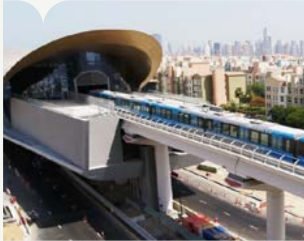
Metro R17 T1T2 Client: Al Yousuf Electronics LLC Brand: Fujitec | Quantity: 02
