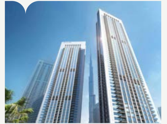
Downtown Views Client: KONE Middle East UAE Brand: KONE | Quantity: 21
