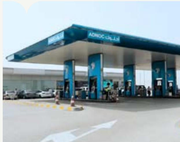
Mazyad Station Al Ain Client: KONE Middle East UAE Brand: KONE | Quantity: 01
