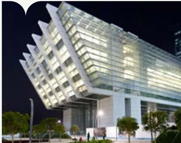
Abu Dhabi Financial Center Phase 2 Client: ThyssenKrupp Brand: ThyssenKrupp | Quantity: 06
