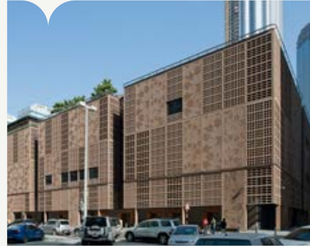
Abu Dhabi Central Market #1 Client: ThyssenKrupp Brand: ThyssenKrupp | Quantity: 03
