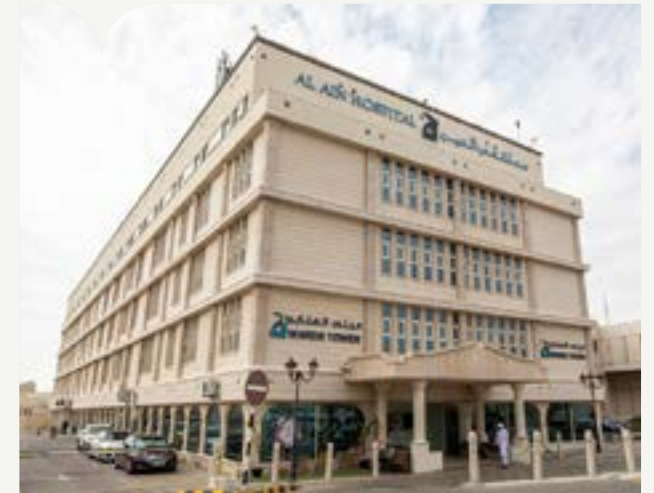
Al Ain Hospital Client: KONE Middle East UAE Brand: KONE | Quantity: 09
