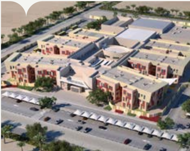
Al Ain Schools Client: KONE Middle East UAE Brand: KONE | Quantity: 02
