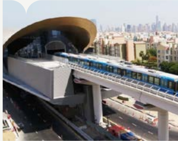
Metro R17 T3T4 Client: Al Yousuf Electronics LLC Brand: Fujitec | Quantity: 02
