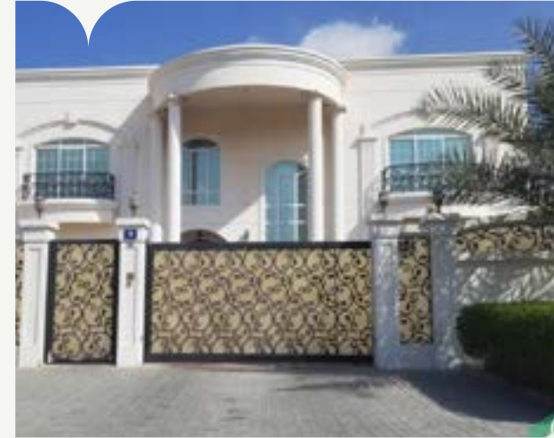
Dubai Barsha 2 Stops Villa Client: Alaa Al Jazeera Elevator & Escalator Brand: Al Sahab | Quantity: 01
