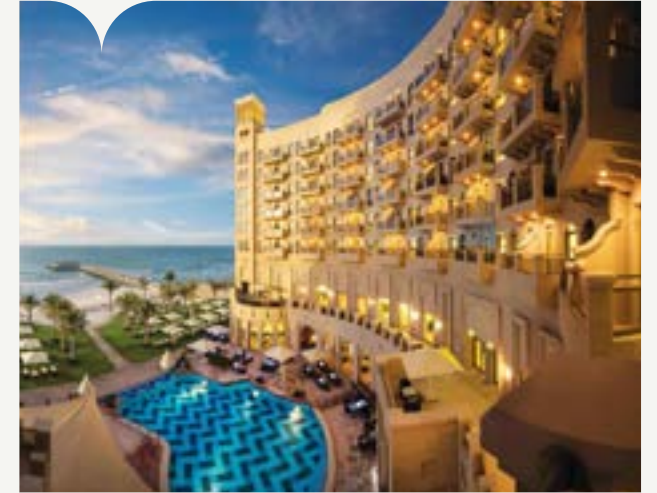
Ajman Palace Villa Client: Alaa Al Jazeera Elevator & Escalator Brand: KINETEK | Quantity: 02
