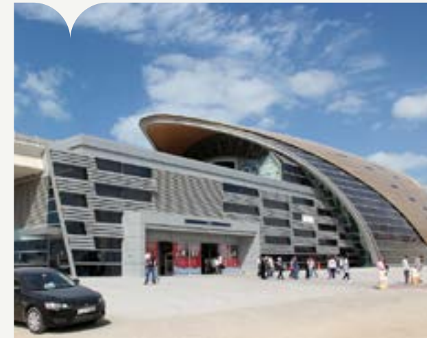
Metro R13 T3T4 Client: Al Yousuf Electronics LLC Brand: Fujitec | Quantity: 02
