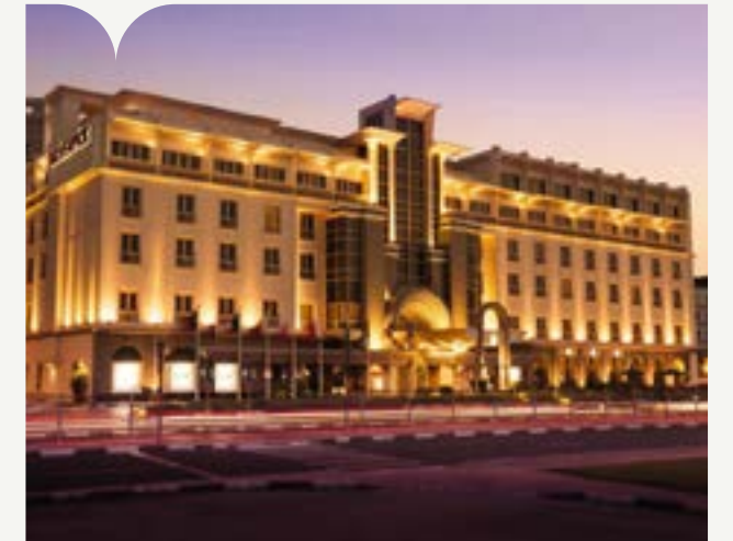
Deira MovenPick Client: Schindler Pars International Ltd Brand: Schindler | Quantity: 12
