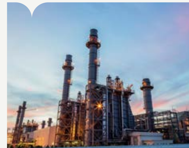
Ruwais Refinery Expansion Client: ThyssenKrupp Brand: ThyssenKrupp | Quantity: 03
