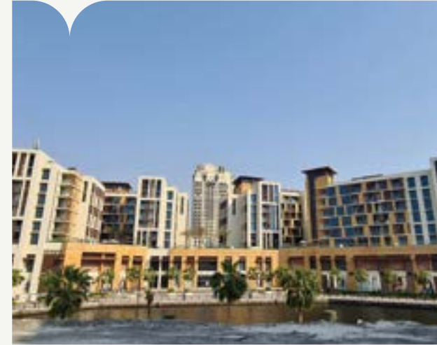
Dubai Wharf Client: KONE / Engineering Contracting LLC Brand: KONE | Quantity: 06
