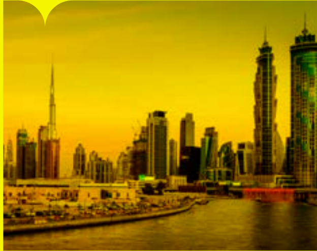
Business Bay 1B Client: ThyssenKrupp Brand: ThyssenKrupp | Quantity: 09
