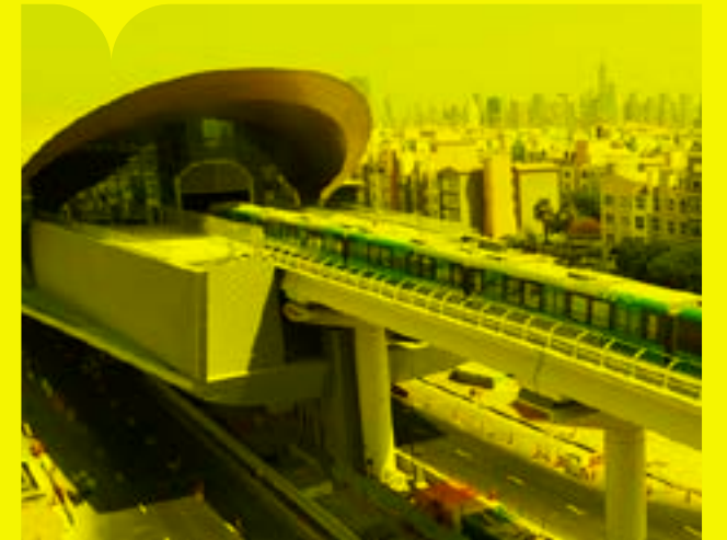
Metro R16T3T4 Client: Al Yousuf Electronics LLC Brand: Fujitec | Quantity: 02
