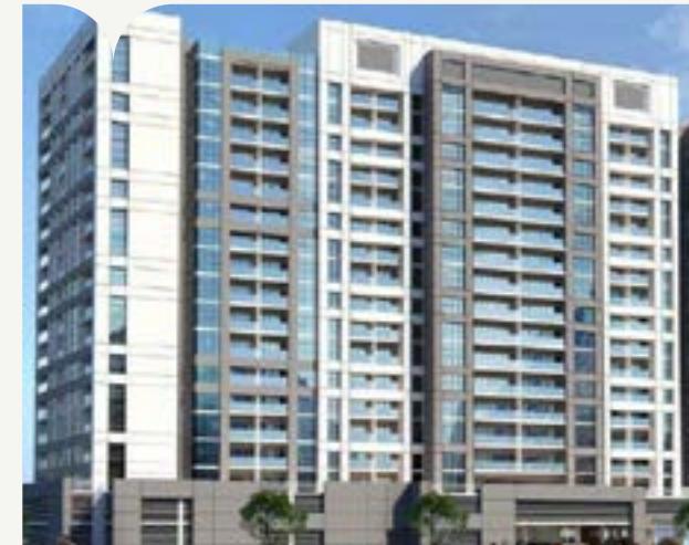
CRC Construction Client: KONE Middle East UAE Brand: KONE | Quantity: 05
