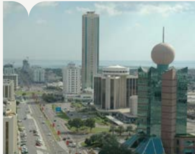
Fujairah Aamar Building Client: Alaa Al Jazeera Elevator & Escalator Brand: Al Sahab | Quantity: 01
