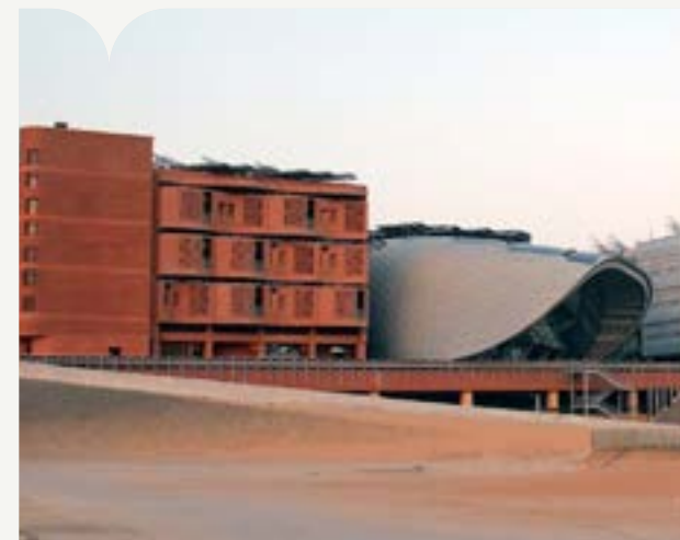
Masdar Institute Client: ThyssenKrupp Brand: ThyssenKrupp | Quantity: 05
