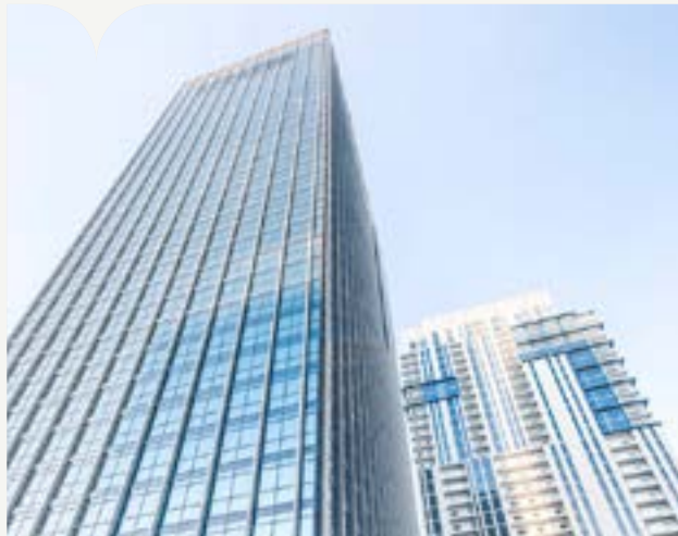
AlRayyan Complex Client: KONE / TERNA S.A - ABU DHABI Brand: KONE | Quantity: 11
