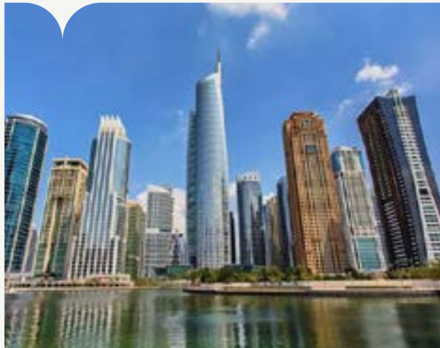
Jumeirah Lake Towers Client: ThyssenKrupp Brand: ThyssenKrupp | Quantity: 05
