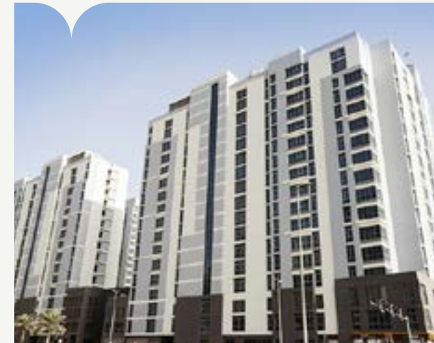
Atlantis Staff Accommodation Client: KONE Middle East UAE Brand: KONE | Quantity: 05
