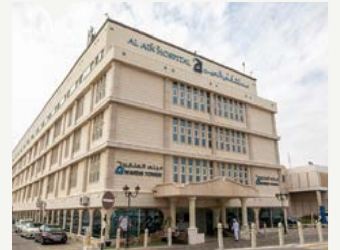
Al Ain Hospital Logistic Building Client: KONE Middle East UAE Brand: KONE | Quantity: 02
