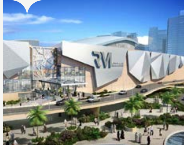
AlReem Mall Client: KONE Middle East UAE Brand: KONE | Quantity: 02
