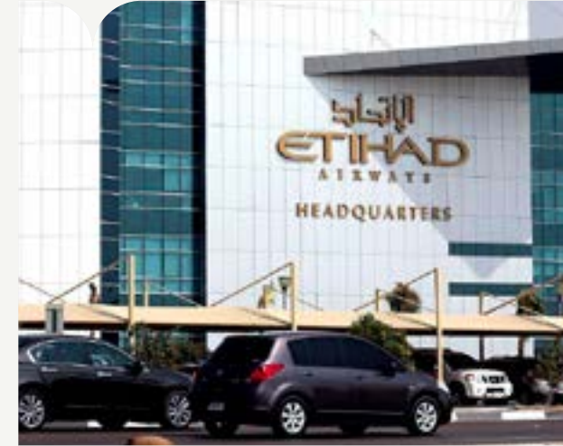
Etihad Complex Client: Schindler Pars International Ltd. Brand: Schindler | Quantity: 02
