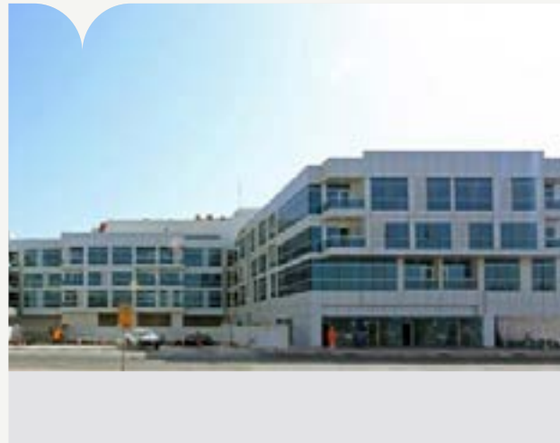
Commercial & Residential Building Client: KONE / Ali Moosa Sons Contracting Brand: KONE | Quantity: 04
