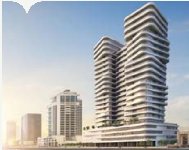
ANWA by Omniyat Client: KONE Middle East UAE Brand: KONE | Quantity: 06
