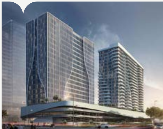
Capital Views Abu Dhabi Client: KONE Middle East UAE Brand: KONE | Quantity: 09
