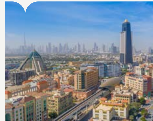
Dubai Health Care Client: KONE Brand: KONE | Quantity: 05
