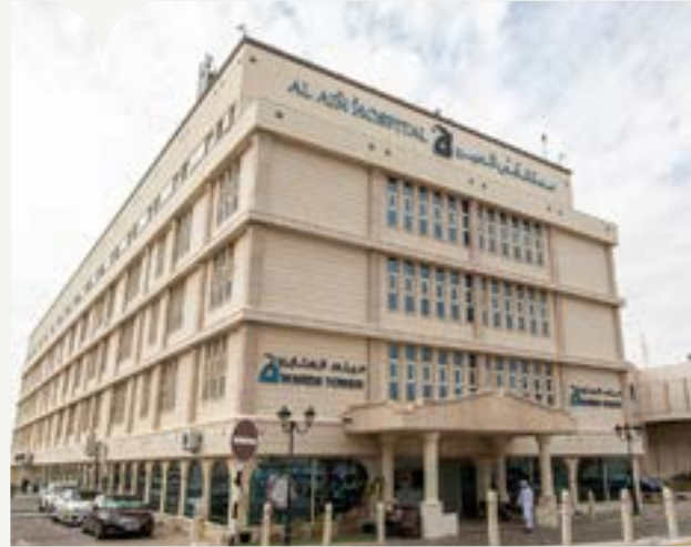
Al Ain Hospital Logistic Building Client: KONE Middle East UAE Brand: KONE | Quantity: 02
